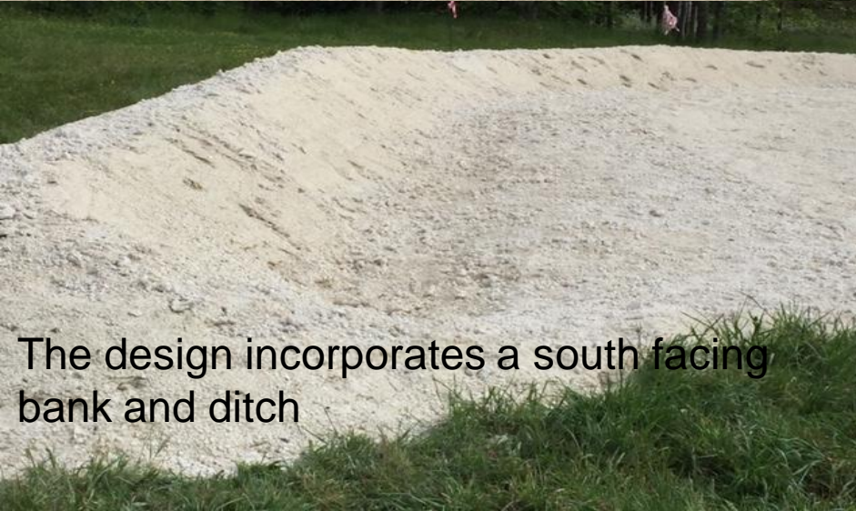
Topsoil is removed and replaced by path grade chalk
